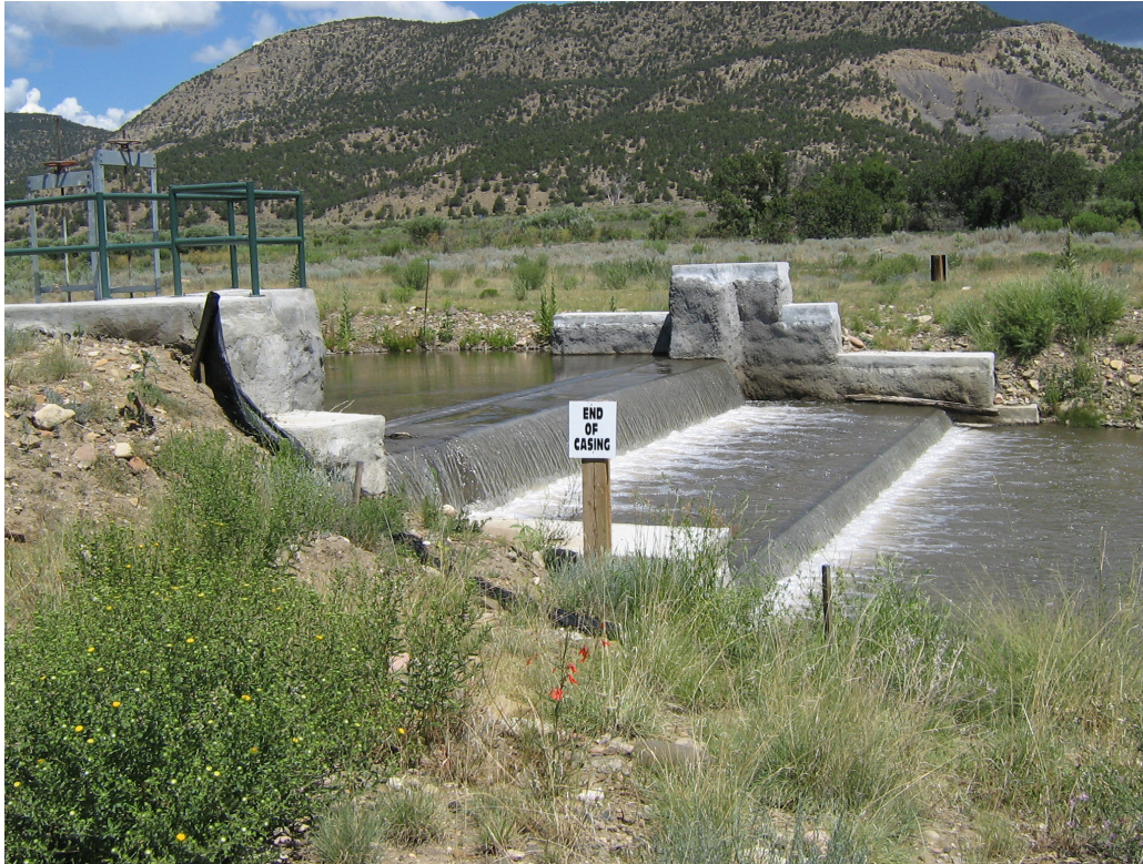
Figure 3 – Cimarron River Diversion Area
