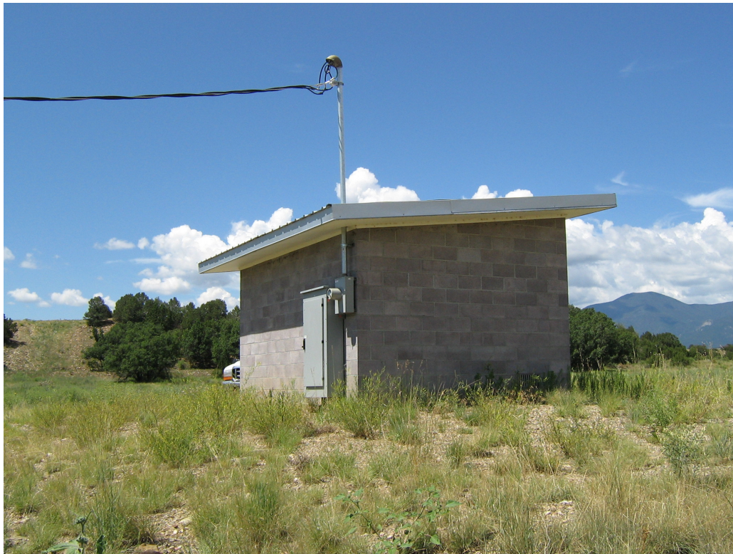
Figure 4 - Cimarron River Pump Station
