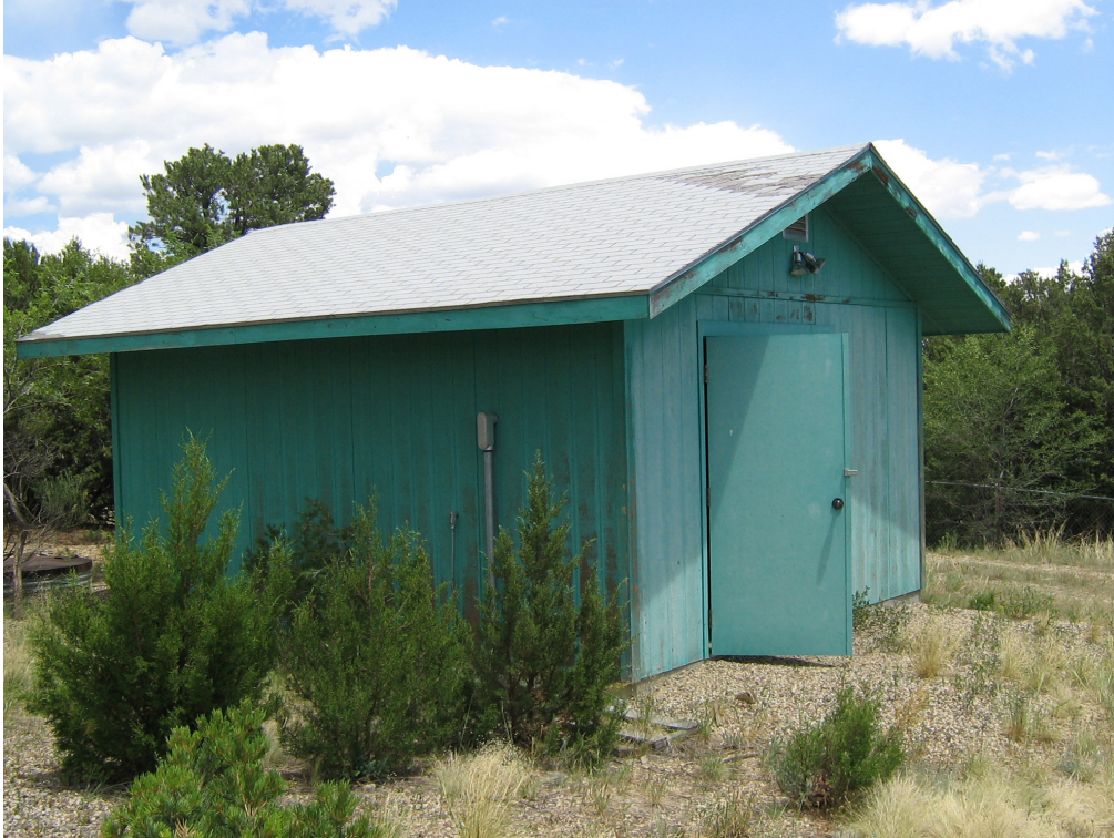
Figure 15 – Lambert Heights Pump Station
