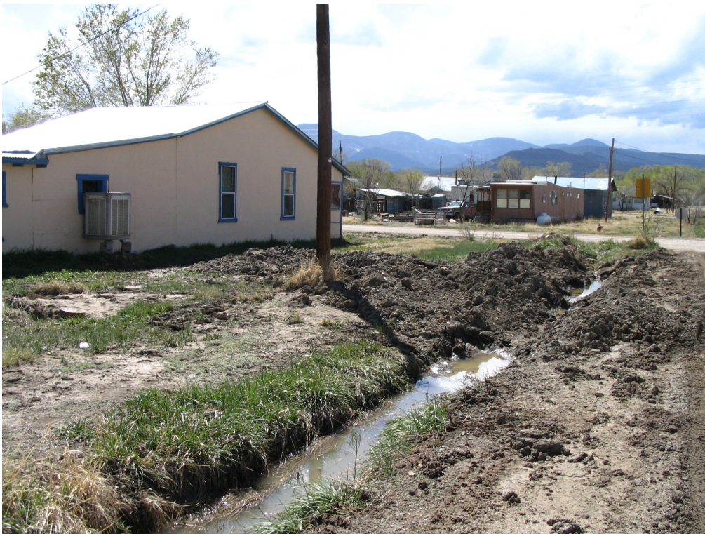
Figure 16 – Damage Caused by Water Main Failure
