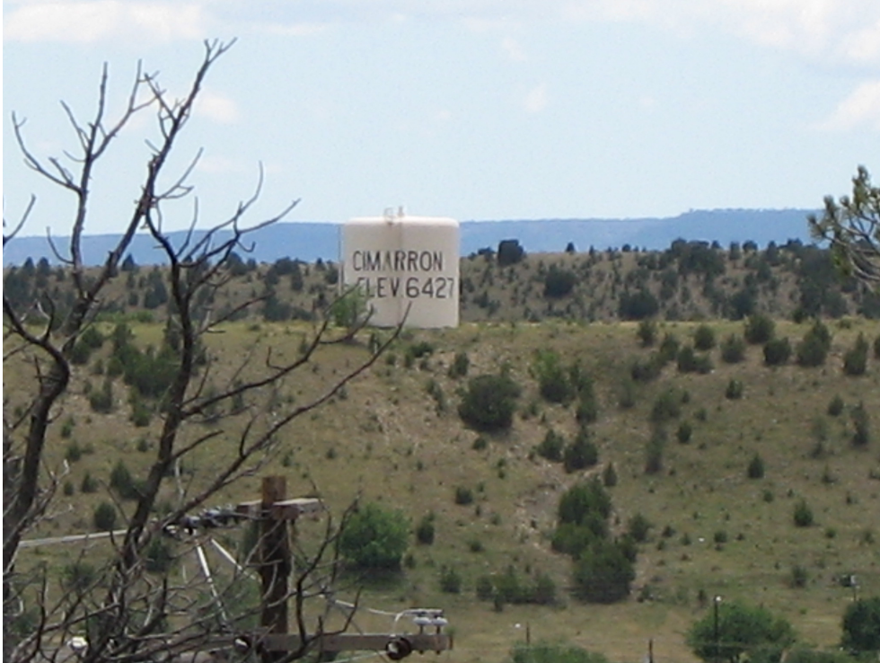
Figure 13 - Cimarron Main Potable Water Storage Tank
