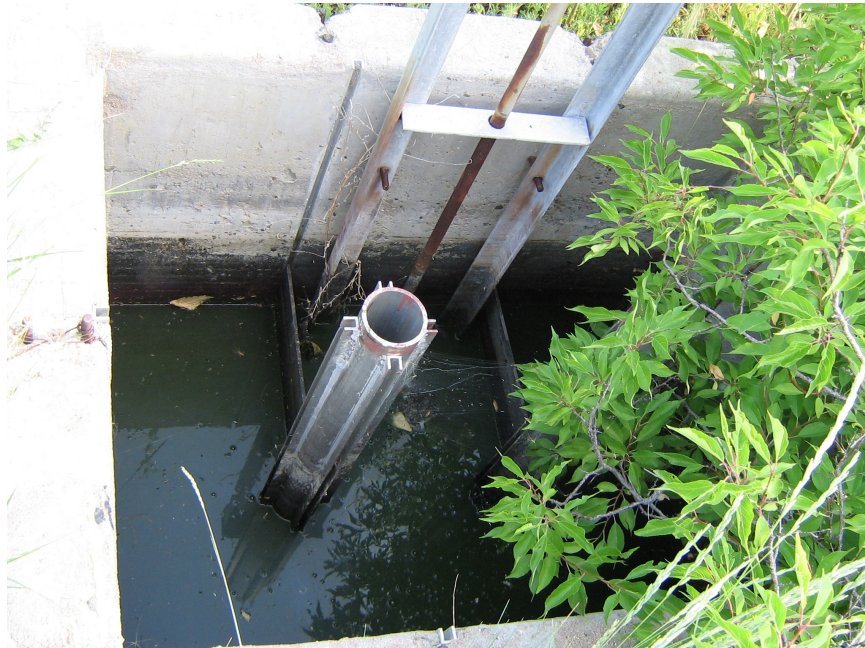
Figure 10 – Effluent Head Gate Detail
