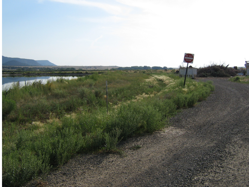
Figure 3 - Access Road Surrounding Treatment Lagoons
