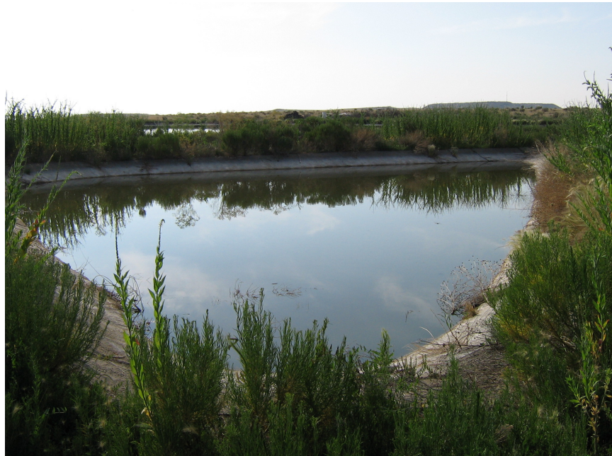
Figure 2 - East Sand Filter Looking North Toward French Lake
