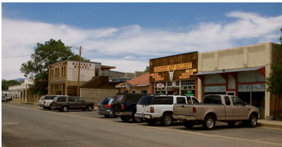
Exhibit III-7: Commercial Uses on Downtown's 9th Street
